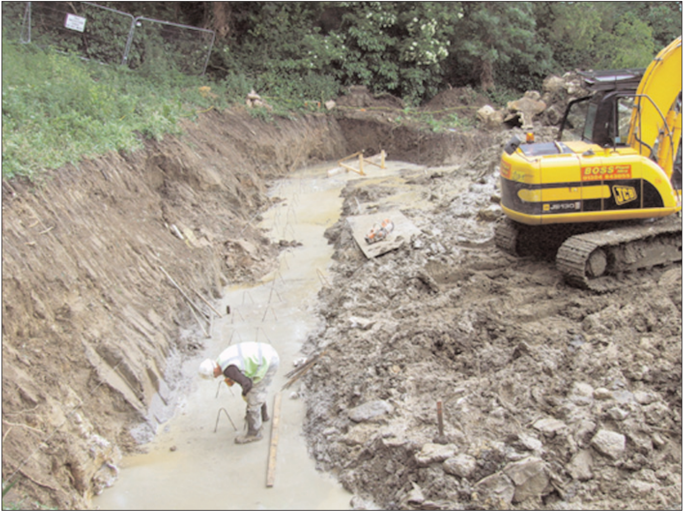
Plate 3. Site Conditions with gushing groundwater and slipping slopes.
