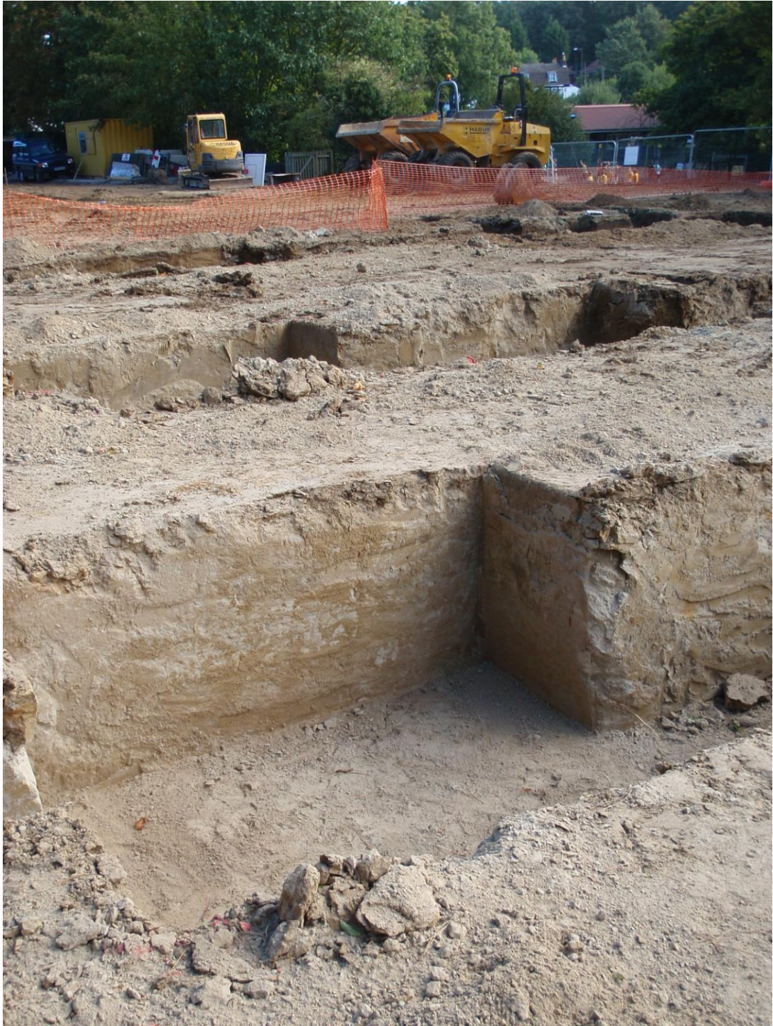
Plate 1. Showing natural geology and foundation trenches for new school
