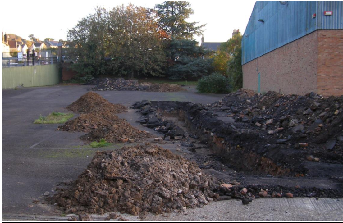
Figure 8: Trenches 1 and 3 (3 in foreground)
