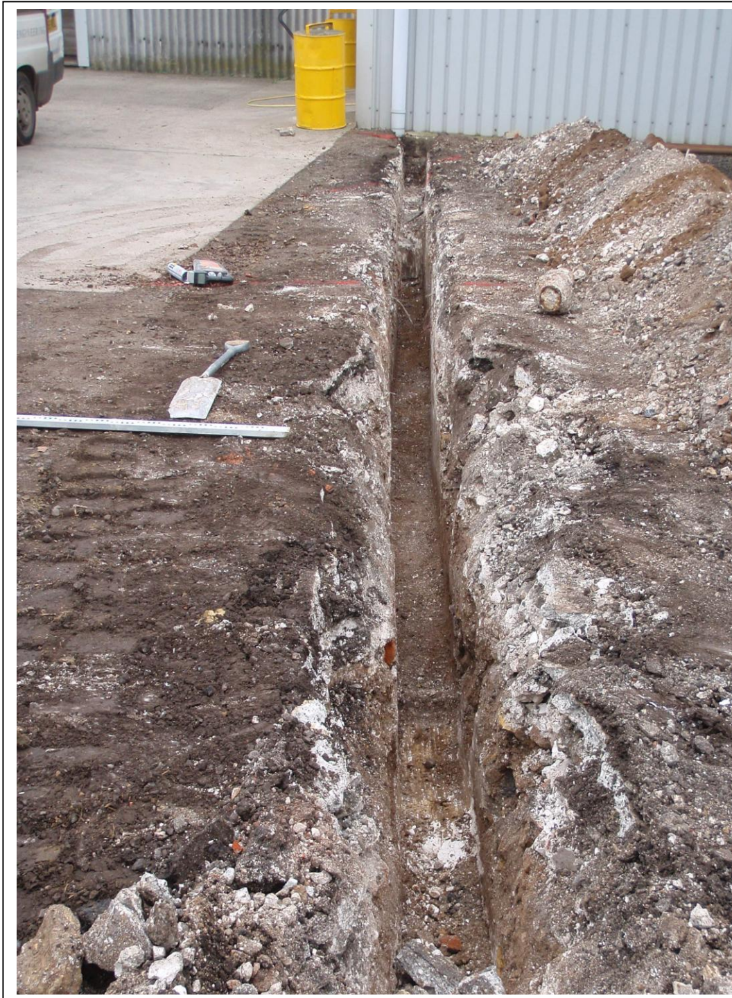
Plate 1. Cable run trench to the main grid hook-up (looking north)
