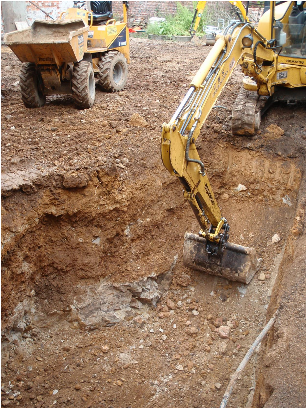
Plate 2. View of excavation for new cellar: facing north
