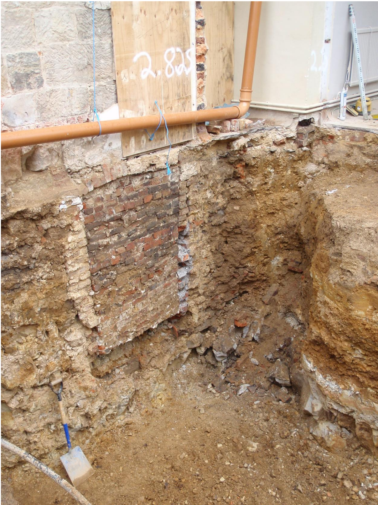
Plate 3. View of existing foundations exposed by excavation for cellar
