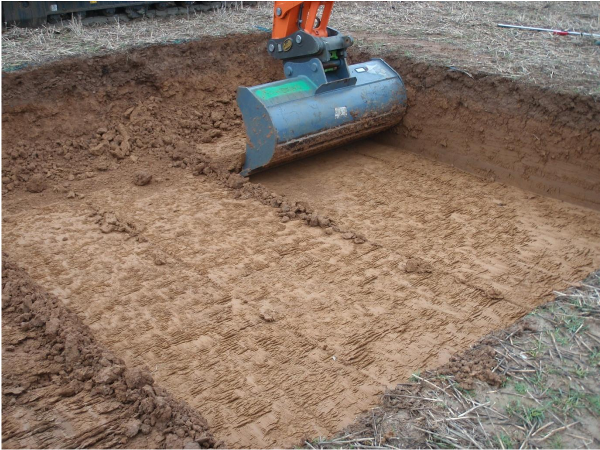
Plate 3. Digging the wind turbine foundation
