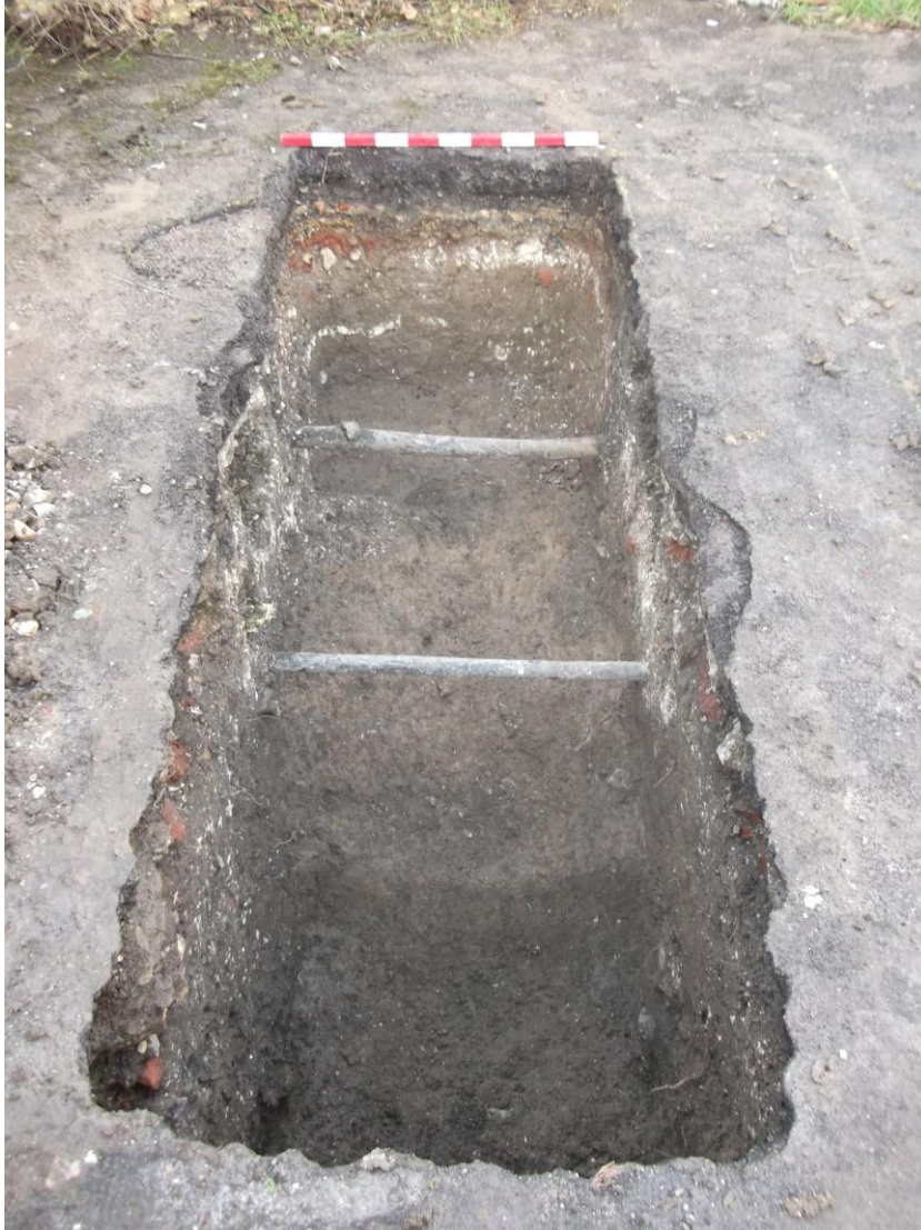
Figure 1 Trench 1 viewed from the south-east
