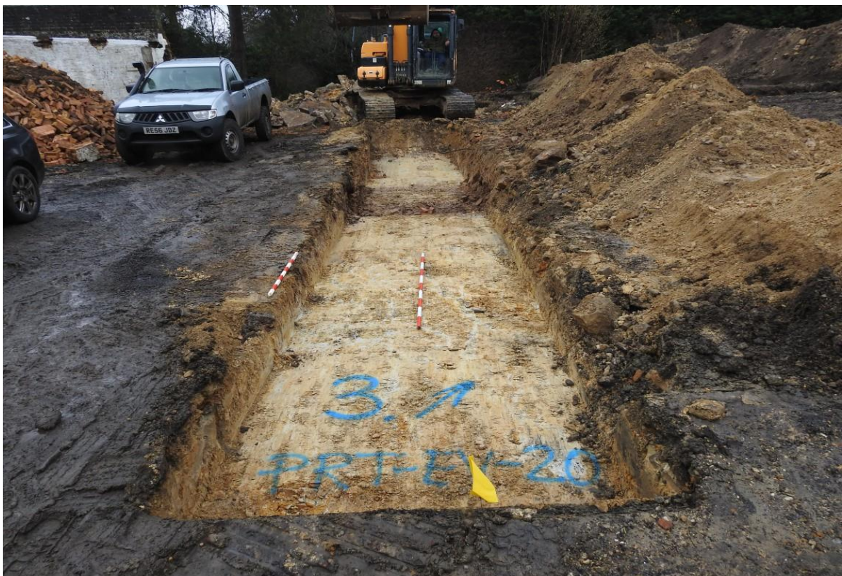
Plate 8: Showing Evaluation Trench 3. Looking north-west with one- and two-metres scales. A collapsed manhole or service duct [303] visible in middle-ground.
