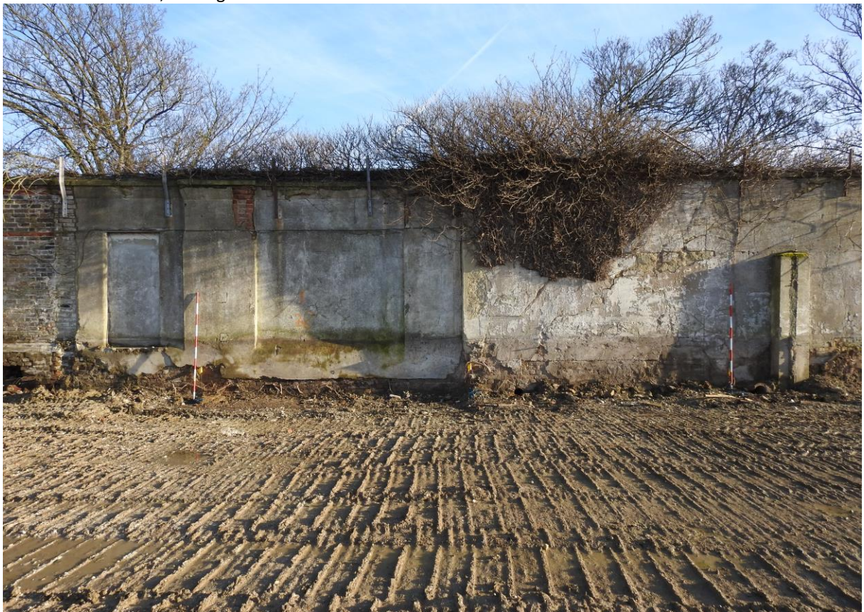
Plate 24: Section J-L, looking south-east with two-metre scales.
