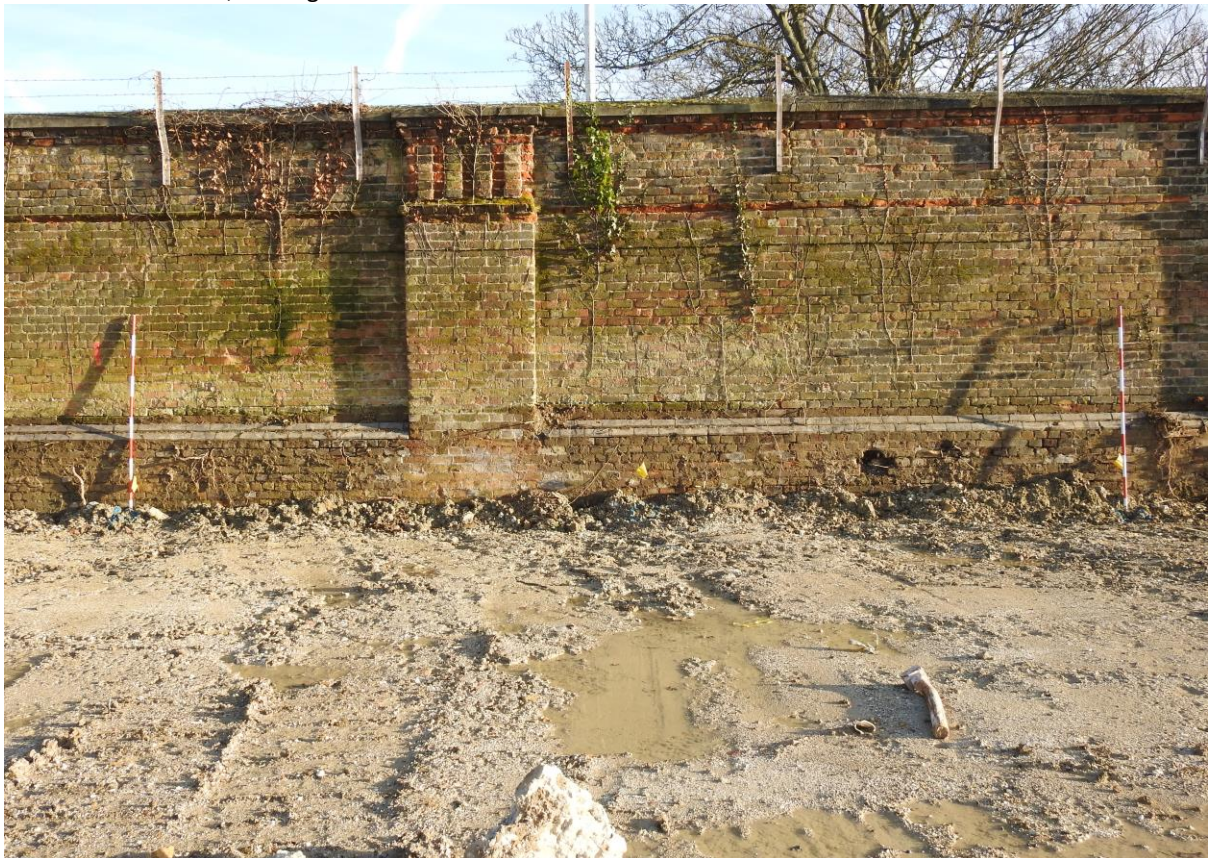
Plate 26: Section N-P, looking south-east with two-metre scales.
