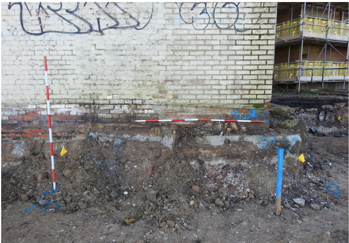
Plate 10: Section X9-X10, looking south with two-metre scales.
