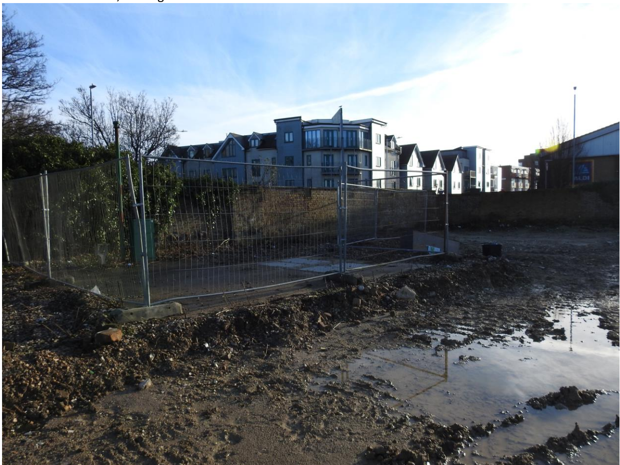
Plate 22: Showing inaccessible area between points G and H. Looking south.
