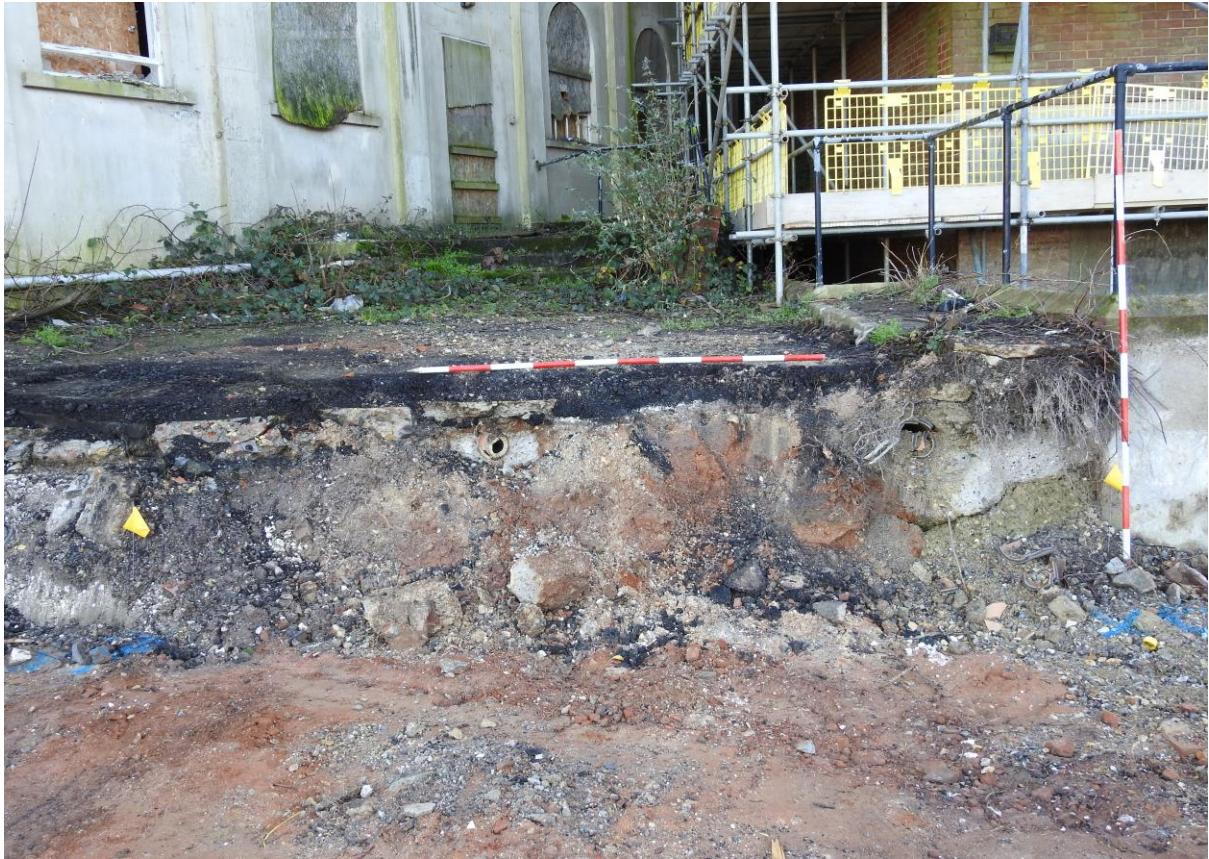
Plate 7: Section X6-X7, looking south with two-metre scales.
