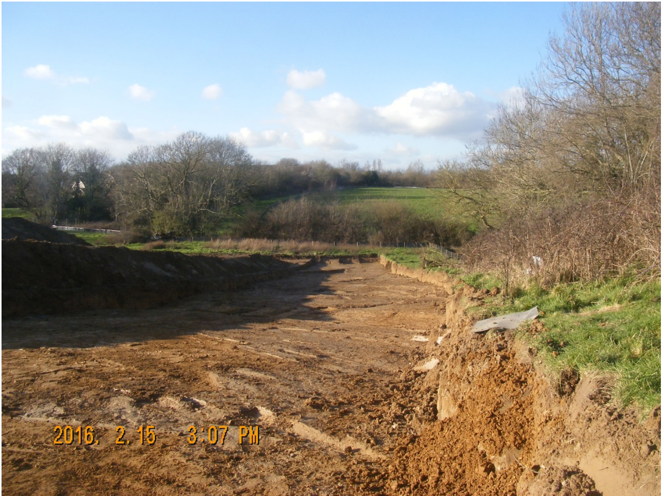
Plate 1: Looking northwest at the area 2 after stripping
