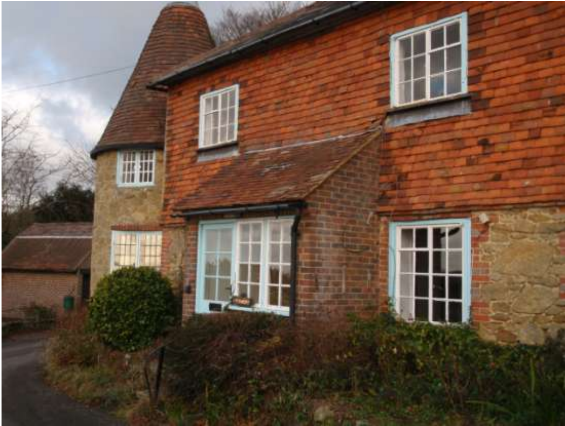
Plate 4. Side view of front elevation (looking west)
