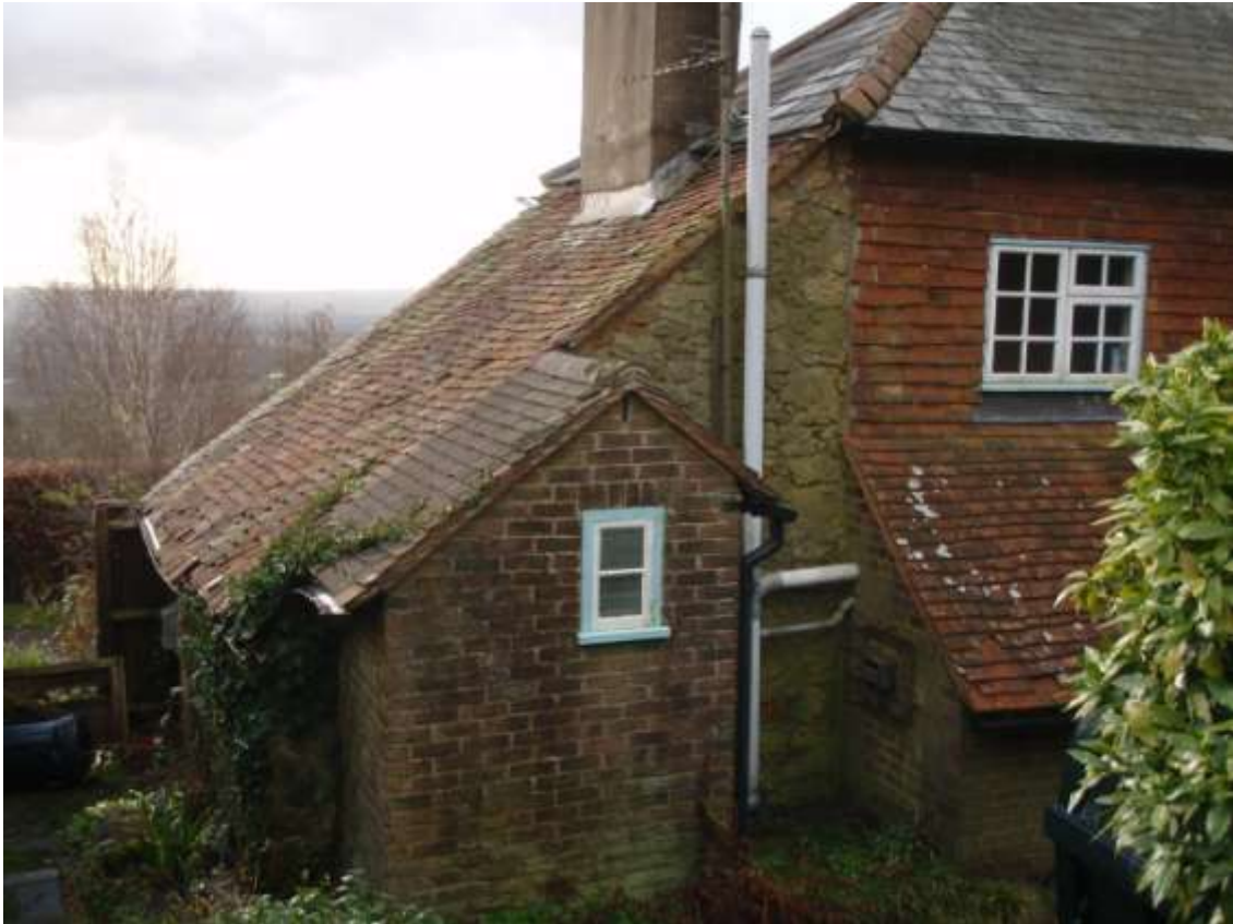
Plate 6. Rear view of kitchen (looking south)
