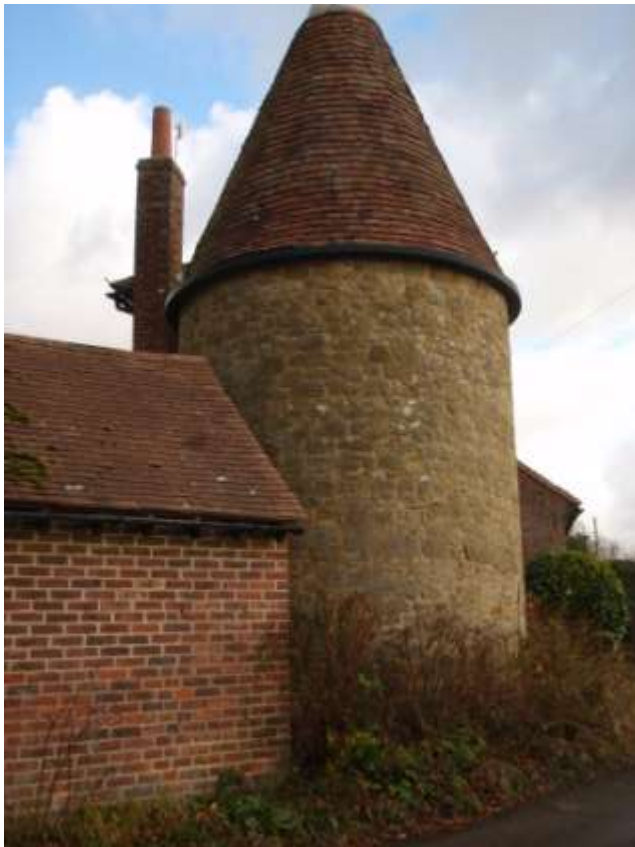
Plate 9. Rear view (looking east) and Plate 10 view of oast (looking NE)
