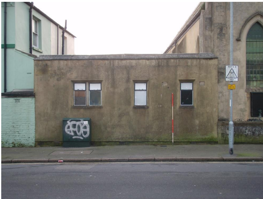
Plate 4. Side view of front elevation (toilets) dating from 1927
