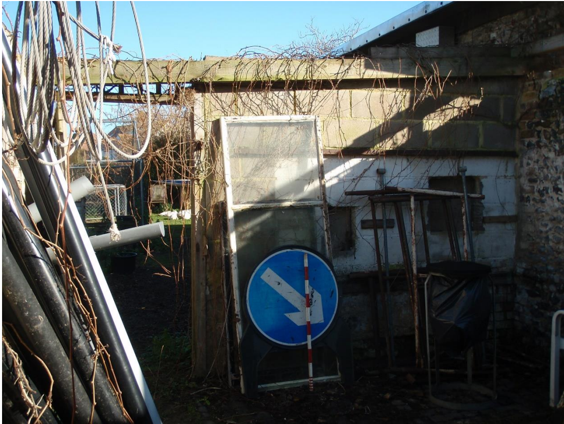
Plate 7. View of internal wall of concrete blocks north end (looking north)
