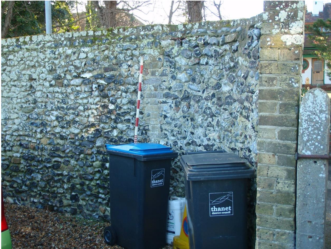
Plate 9. External view of south wall (looking north)
