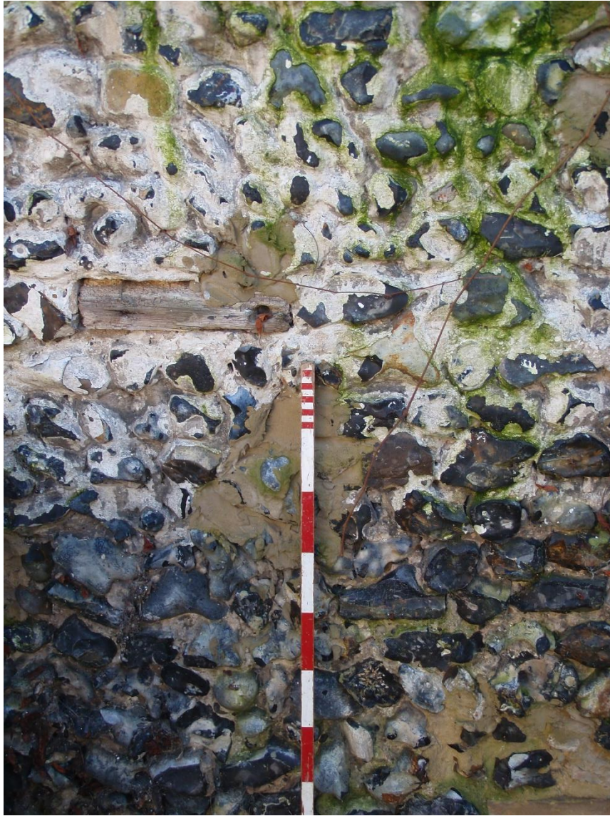
Plate 13. Close up of flint work wall north-east elevation
