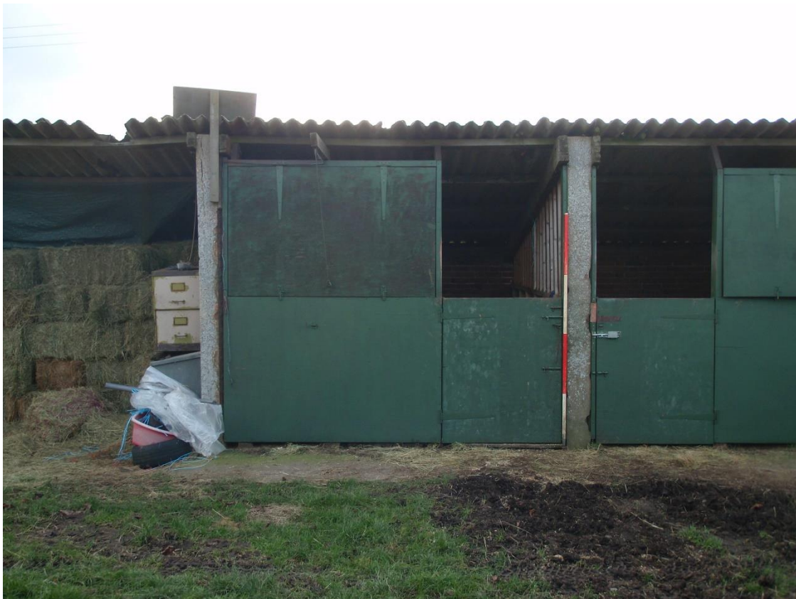
Plate 8. View of Building 'B' (Elevation F) looking SSW
