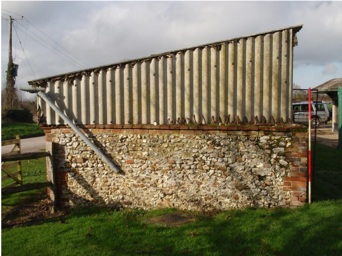
Plate 9. View of Building 'B' (Elevation c) looking NNW
