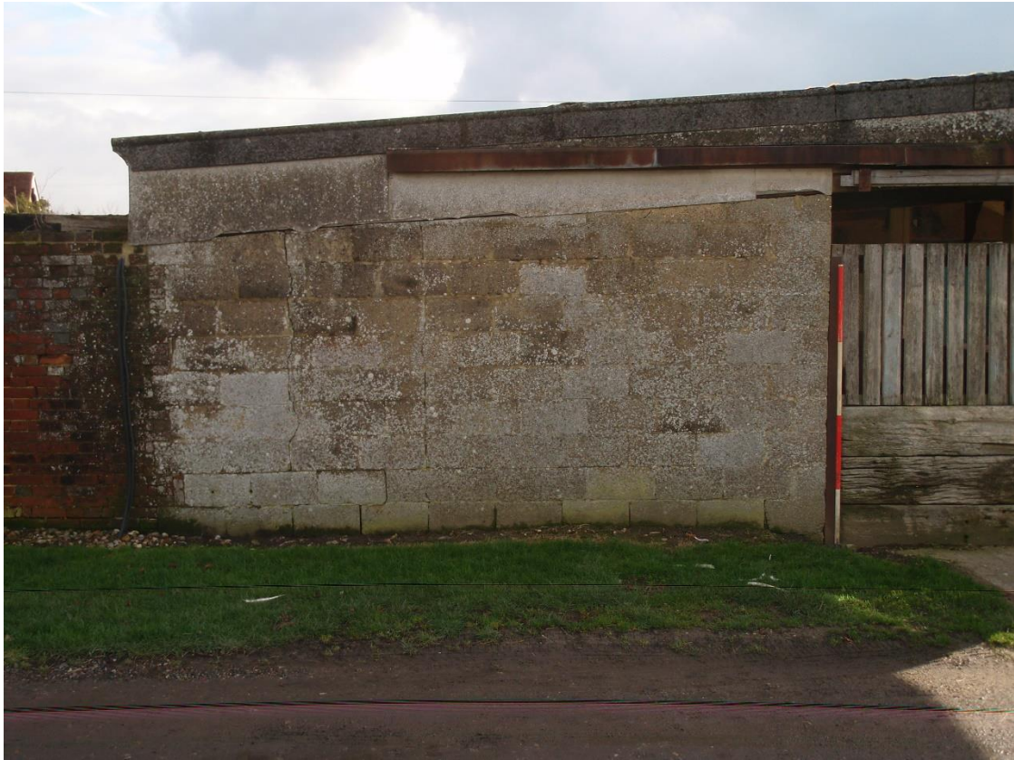
Plate 1. View of external west wall Building 'A' (Elevation A) looking east
