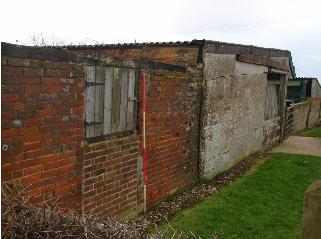
Plate 12. View of Building 'A' (Elevation A) looking south
