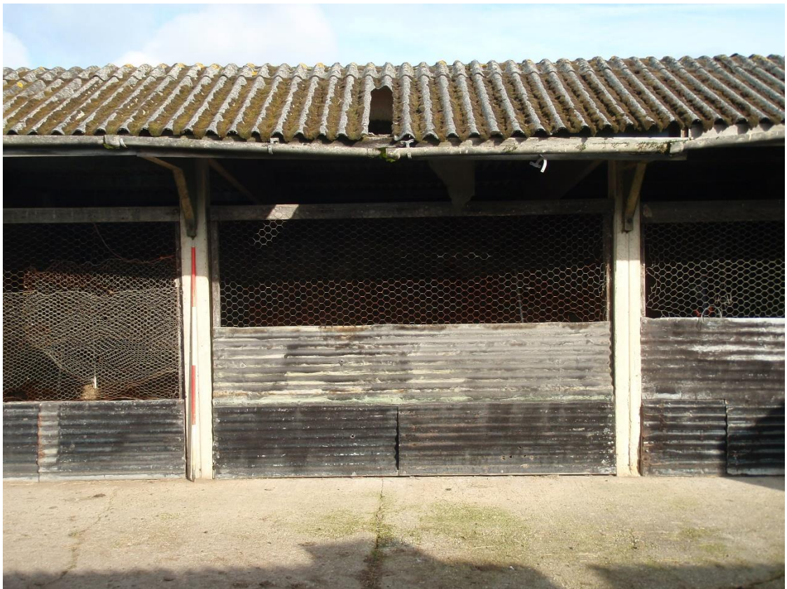
Plate 4. View of Building 'A' (Elevation E) looking NNE
