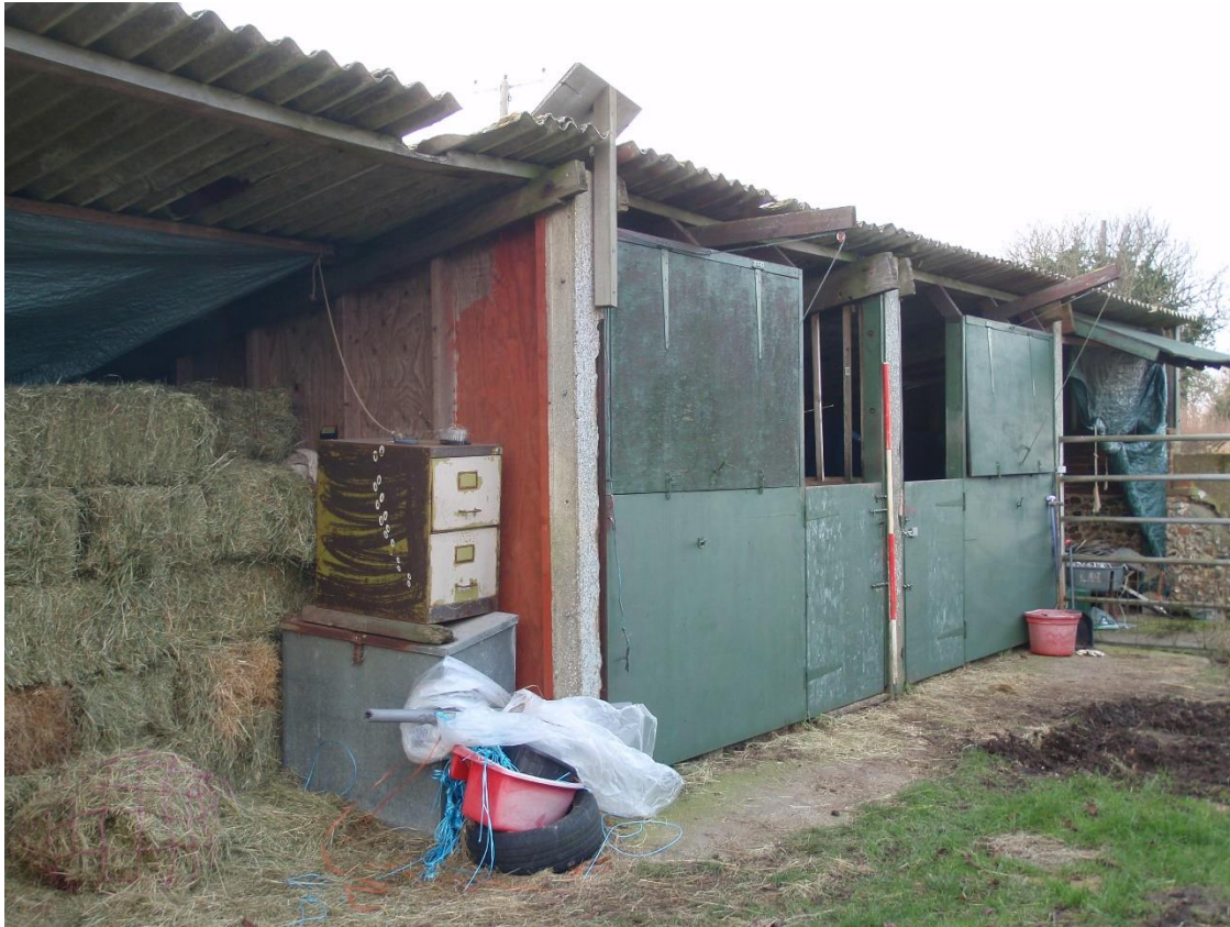
Plate 7. View of Building 'B' (Elevation F) looking south-west
