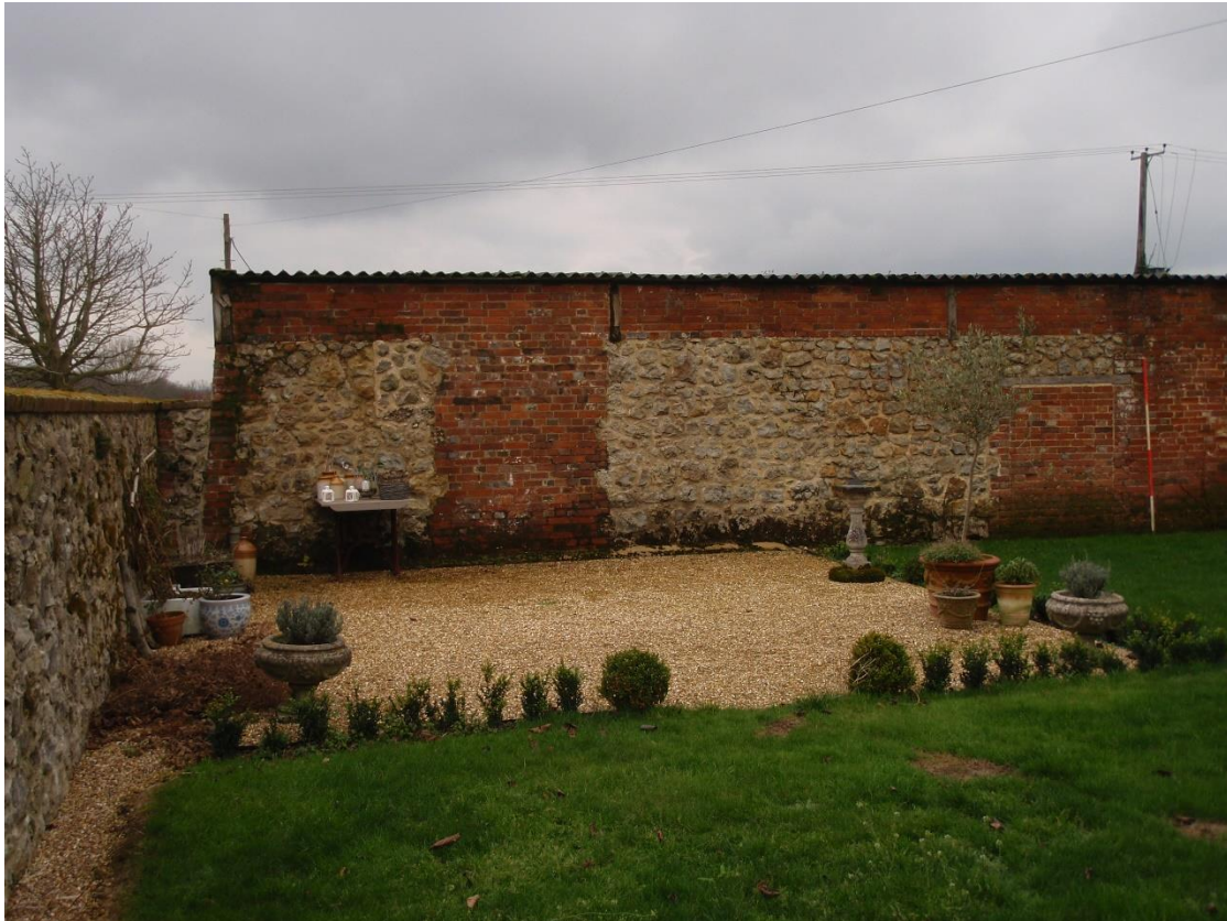
Plate 13. Rear of Building 'A' looking SSW
