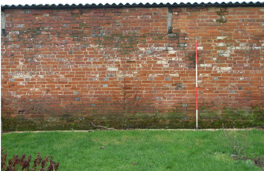
Plate 14. Rear of Building 'A' looking SSW
