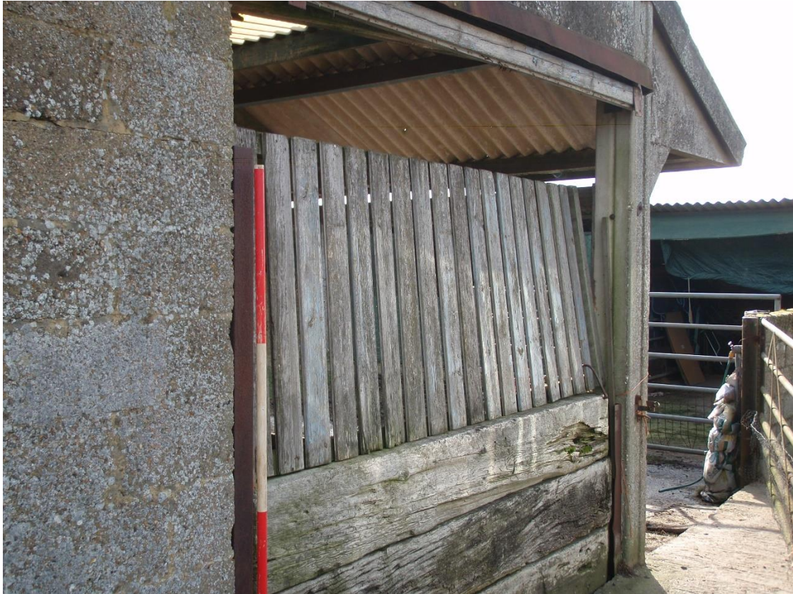
Plate 2. . View of external west wall Building 'A' (Elevation A) looking south-east
