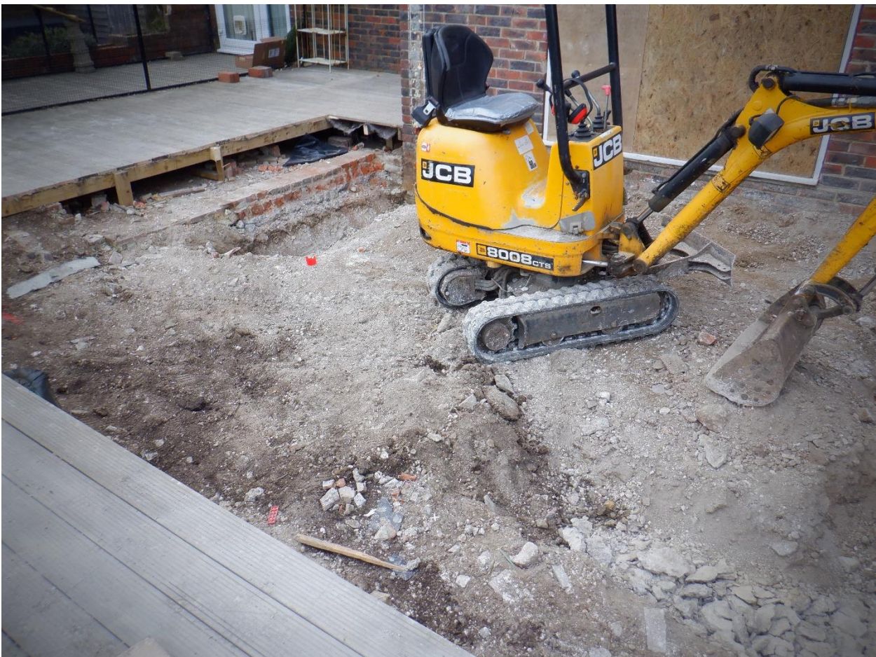
Plate1. Removal of internal concrete floor
